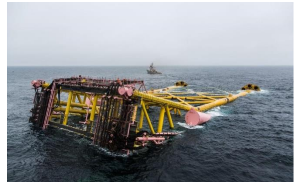
Jacket installation on the Gina Krog field (July 2015)
